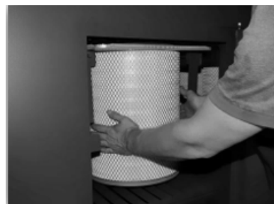
3. Slide filter cartridge(s) out
